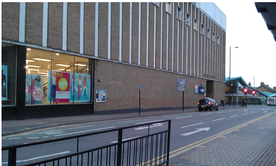
Plate 2 – Heygate Avenue/Alexandra Street
